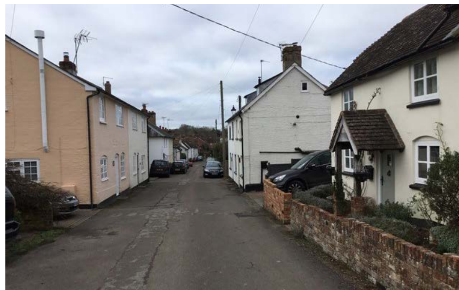
View westwards along West Street
