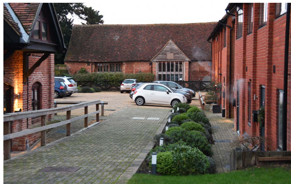
The Cross Barn, Palace Gate Farm, seen from the High Street
