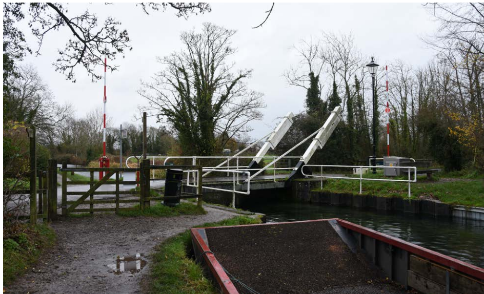
Swing Bridge over the canal
