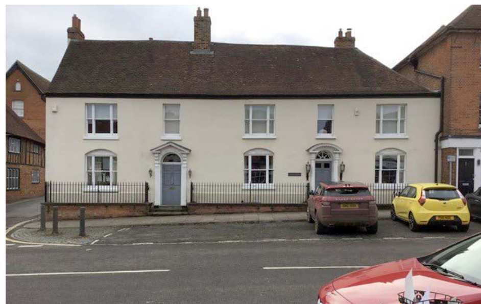
Nos. 67-69 High Street. The re-fronted north façade of a major 15th-century courtyard house
