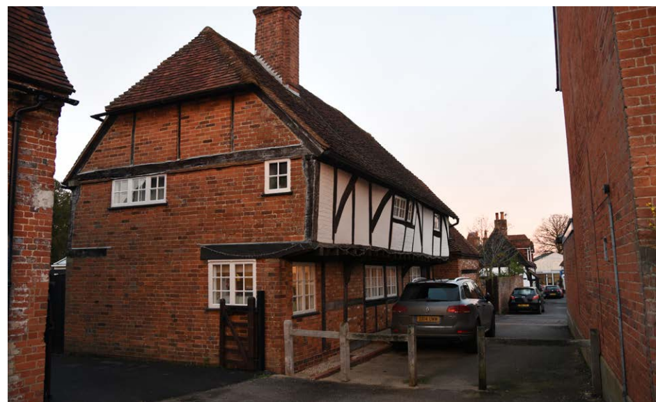
View of Stoney Cottage from the Bury
